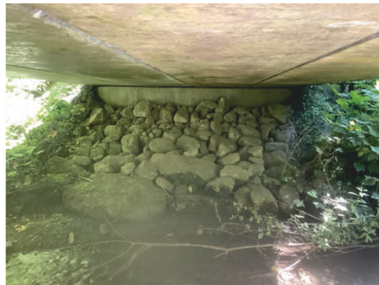
Right Bank Abutment when facing downstream
