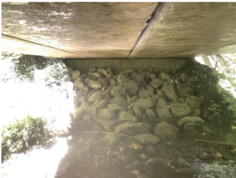
Left Bank Abutment when facing downstream
