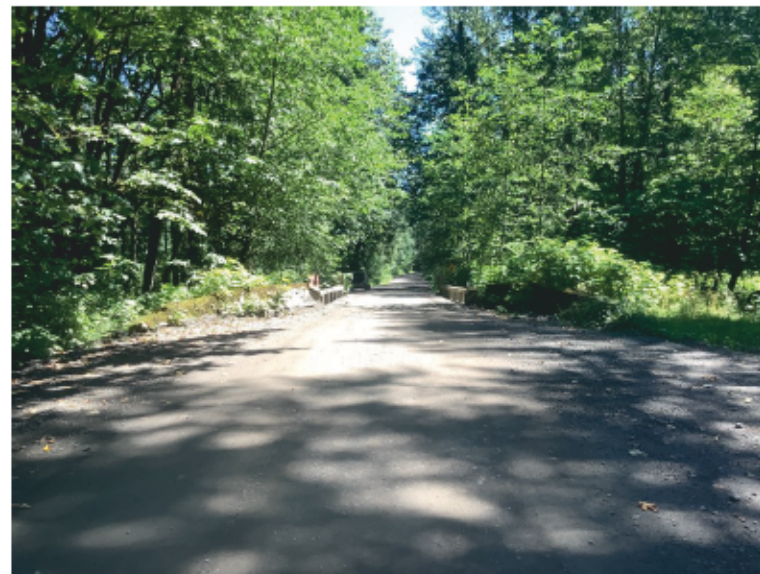
Approach from Left Bank when facing downstream
